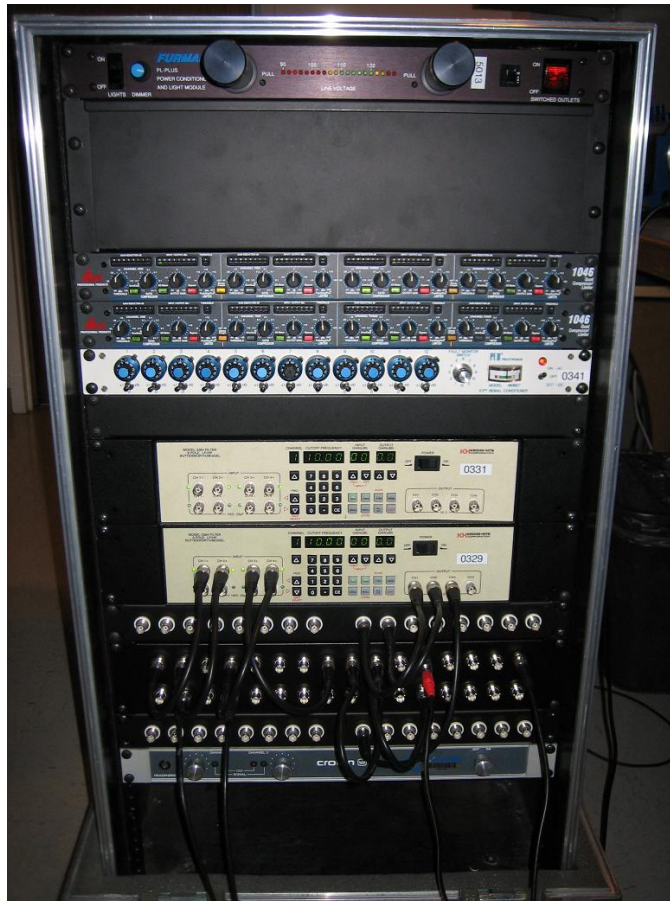
Figure 3.3 The Rack Setup
